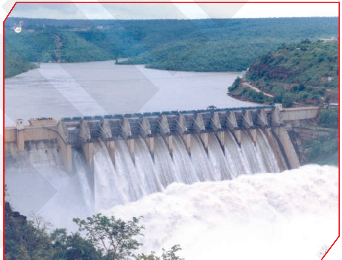
Bhakra Nangal Dam
